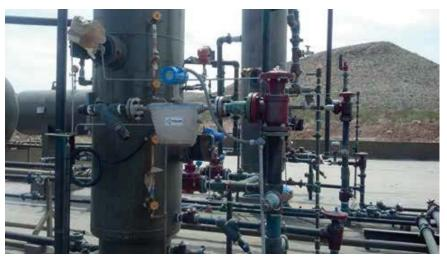
A Tricor Coriolis flowmeter measuring water coming off a separator. (Photo courtesy of AW-Lake)
