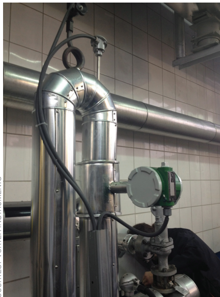
Inline wafer multivariable vortex flowmeter used to measure steam at a soap and detergent manufacturing facility in Poland.
